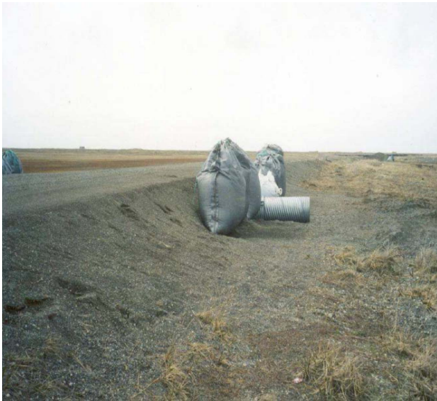
Photo 3: Material washed out of the roadbed by rising waters of Marryat Inlet, 2006.
