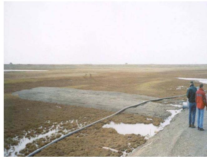
Photo 4: Road embankment at the point of the washout, 2006.
